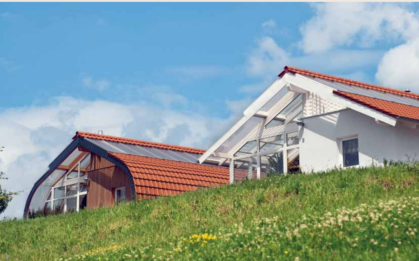
Onion shape or gable roof – the bio-solar house functions almost entirely without technology, and saves energy too.
