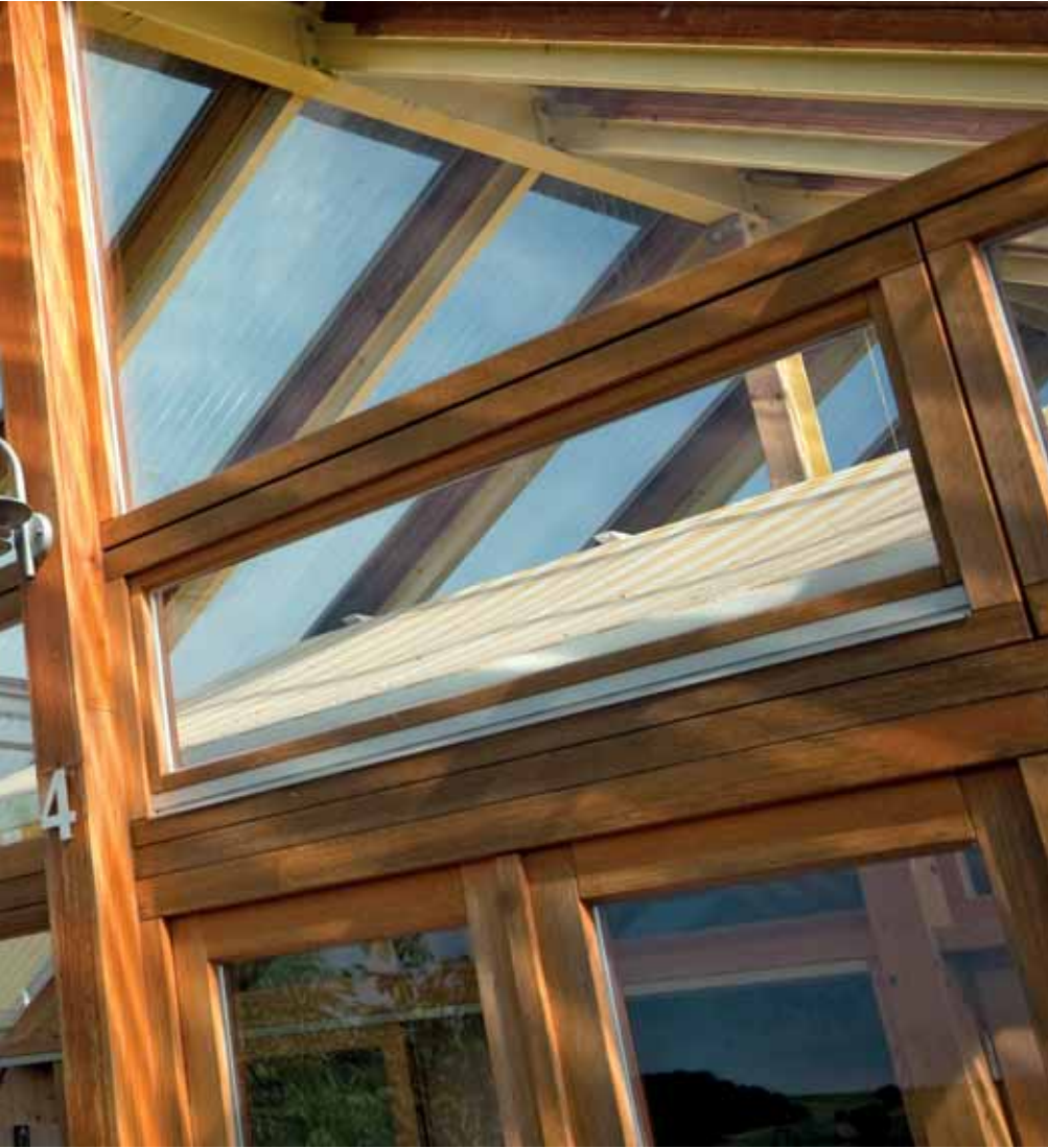
Air flaps in the roof let hot air escape in summer and keep the inner house nice and cool.
