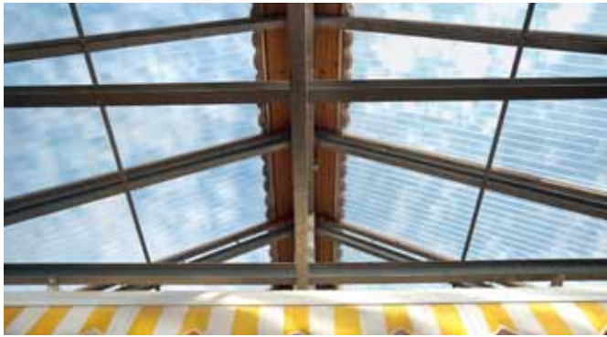
Transparent multi-skin sheets provide the positive greenhouse effect.
