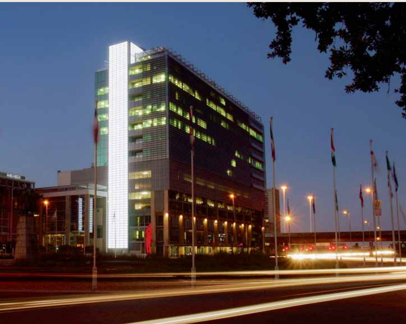
Almost an established sight in the city: The impressive light strip at Cape Town International Convention Centre is made of 1,700 ACRYLITE® sheets.
