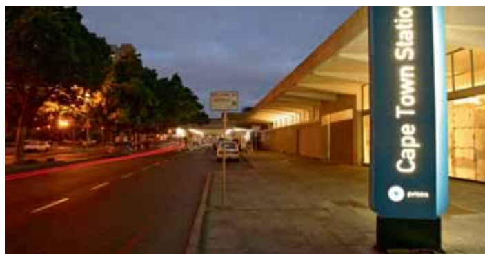
Highlights at the main station: an ACRYLITE® light strip runs round the upper story of the main building at a height of almost seven feet. It shows travelers the way, with the help of numerous illuminated signs.
