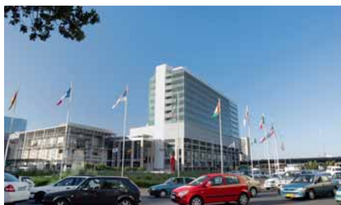
The convention centre is located at a traffic junction. To avoid dazzling drivers, the facade must not reflect the sun.
