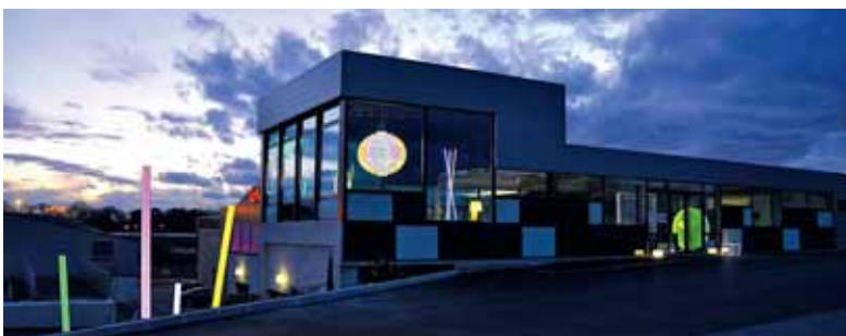
The showroom in Biarritz, France. It's clear looking in from outside that light is the dominant element there, as decoration, exhibit and signpost.
