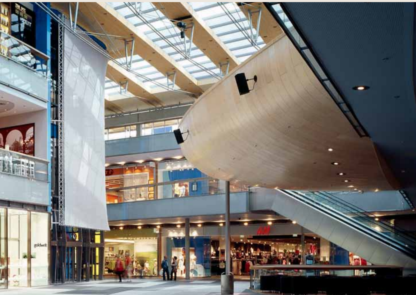
Holder of an award as the world's most sustainable shopping center: "Atrio" in Austria. Geothermal energy is obtained from 652 glowing piles beneath the building. Since shopping malls usually cover large surface areas, they are very suitable for this type of energy generation.
