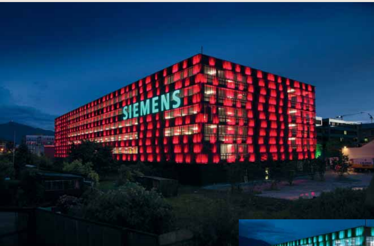
Siemens has changed track: instead of fluorescent tubes, the logo is now lit by energy-efficient LEDs. To achieve the same color effect and luminosity with the light-emitting diodes, the material had to be perfectly adjusted to the LEDs.
